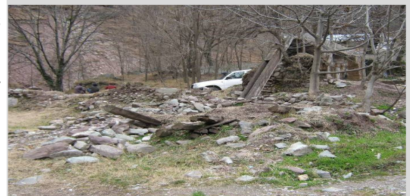
Destroyed water mill in Kewai union council, Mansehra
